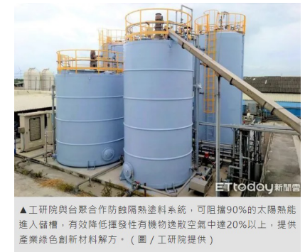
The Industrial Technology Research Institute (ITRI) collaborates with USI on 'cooling' coatings, which can block 90% of heat and reduce the emission of volatile organic compounds by 20%.
