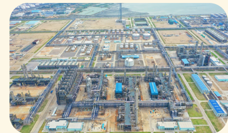
Aerial view of the steam cracking unit
