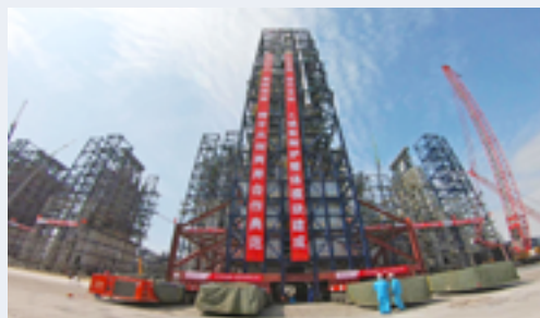
▲ Turnkey transportation and installation of the ethylene cracking furnace.
