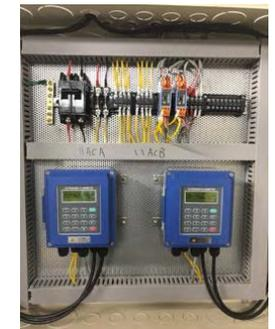
Chiller Flow Meter and Digital Electricity Meter System
